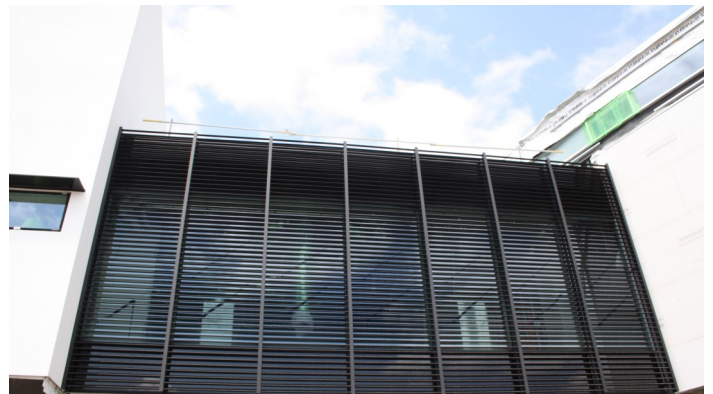
External louvres will filter light.
