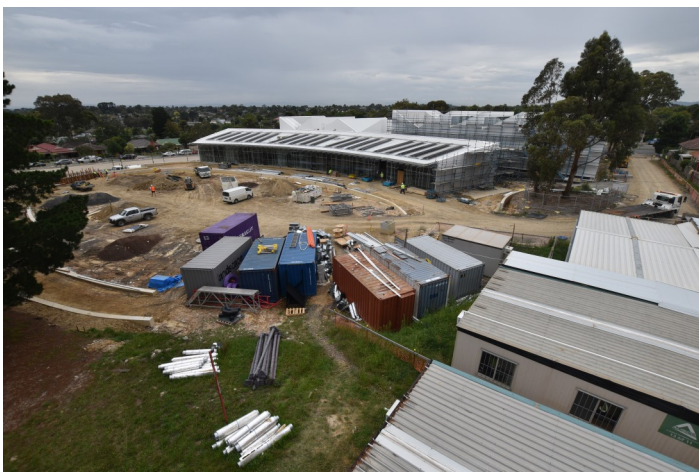
Aerial view of north perspective of site.
