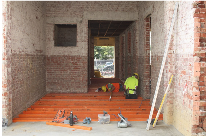
Substrate flooring being laid in heritage building.
