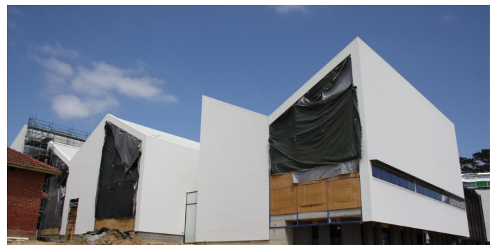
Large frittered glass will be installed on the east side.
