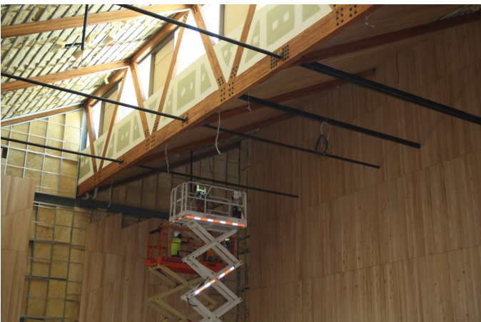
Installing large wooden panels in the stadium.
