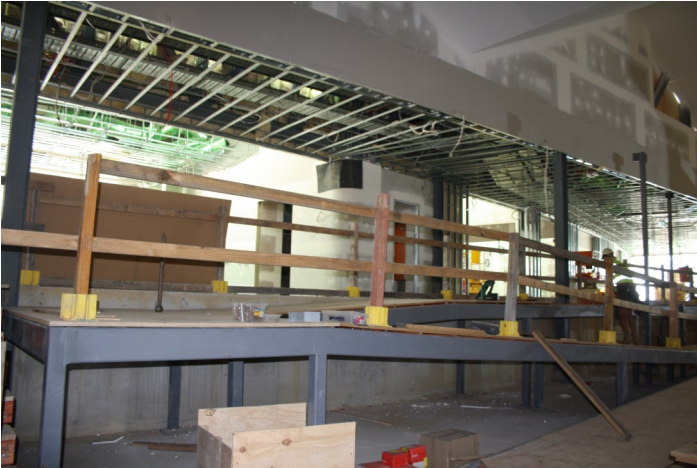
A large accessibility ramp connects the levels.
