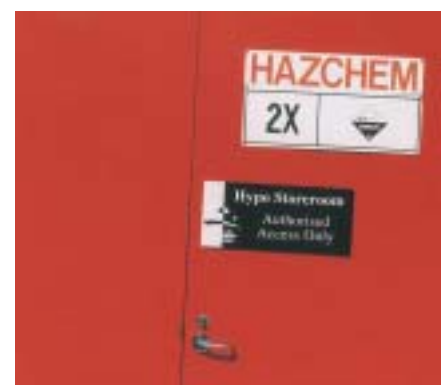
Figure 2 Hazchem signage for packaged dangerous goods
