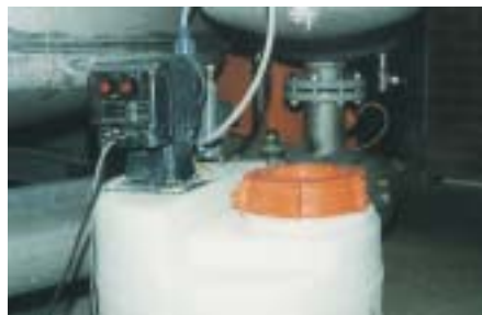
Metering pump mounted on liquid container
