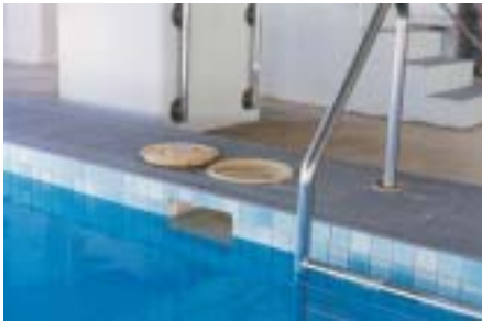
Figure 27 Skimmer box and lint trap
