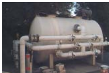
Figure 29 Medium rate pressure filter for larger pool
