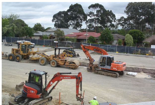
Car park works underway
