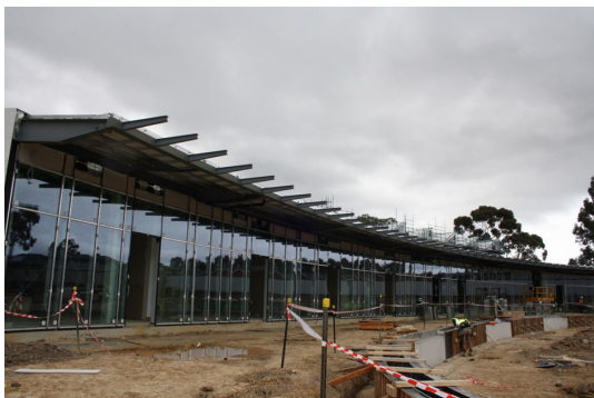
A concrete retainer wall shapes a large outdoor passive leisure area.
