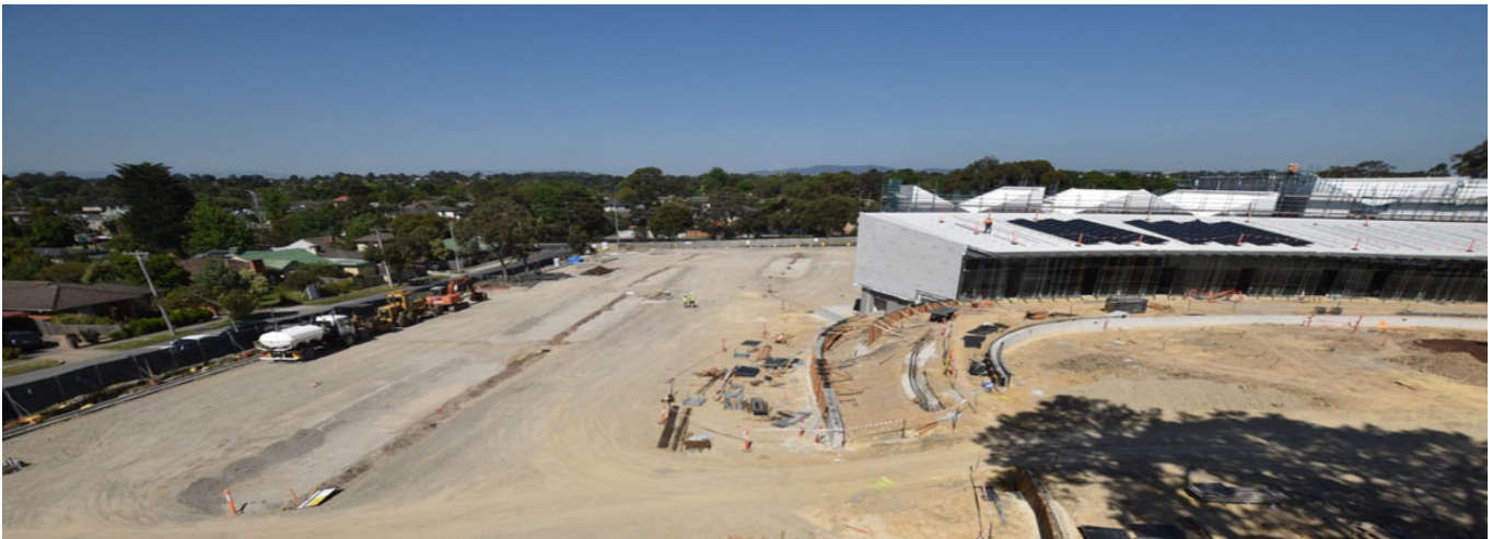
Aerial view of north perspective of site.
