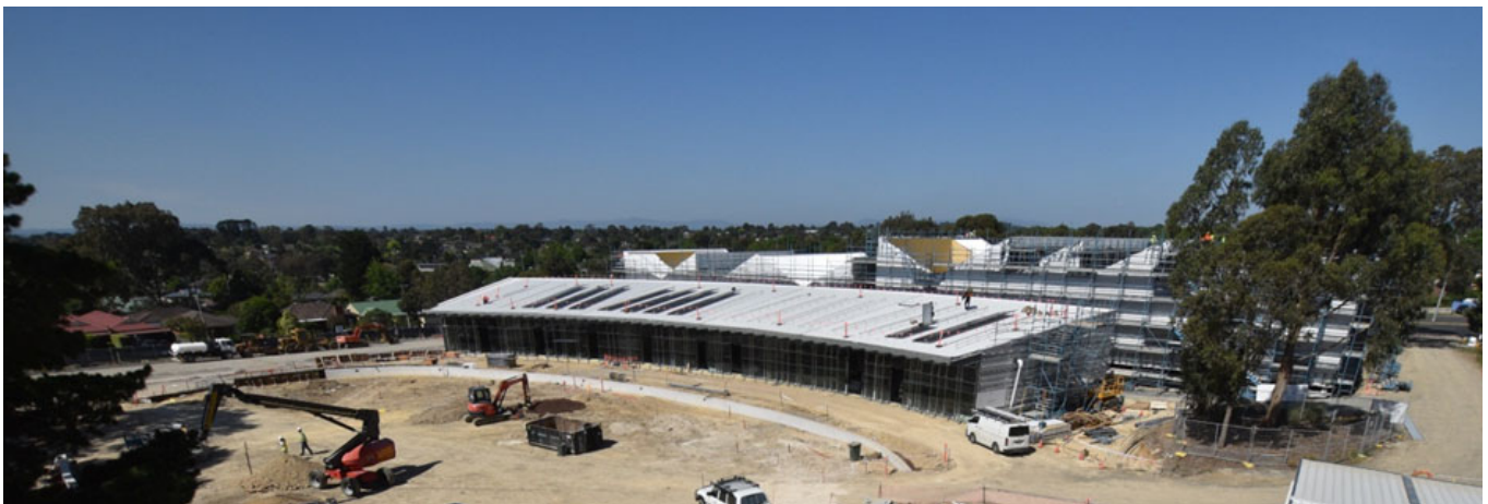
Aerial view of west perspective of site.
