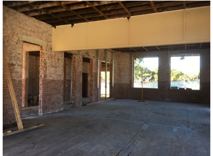
Preparation works continue for complete restoration of the heritage building.
