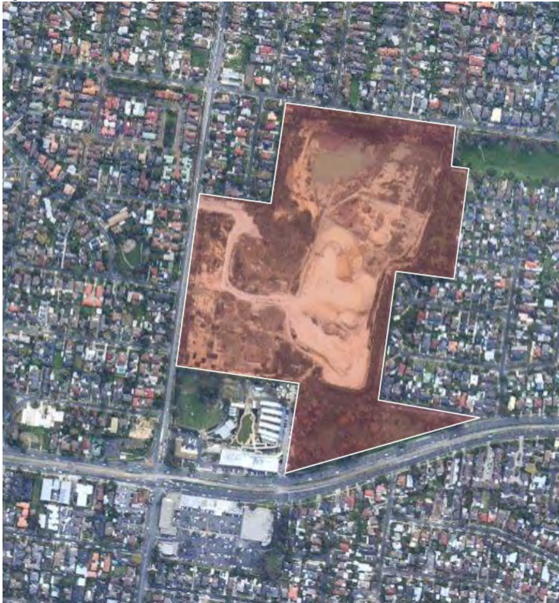
Figure 1 – 78 Middleborough Road, Burwood East
