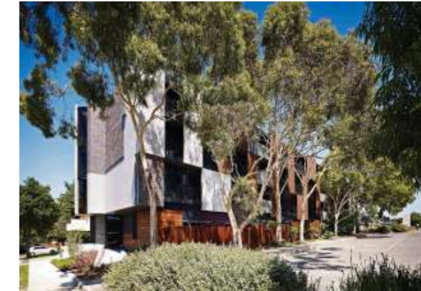
External view of the building
