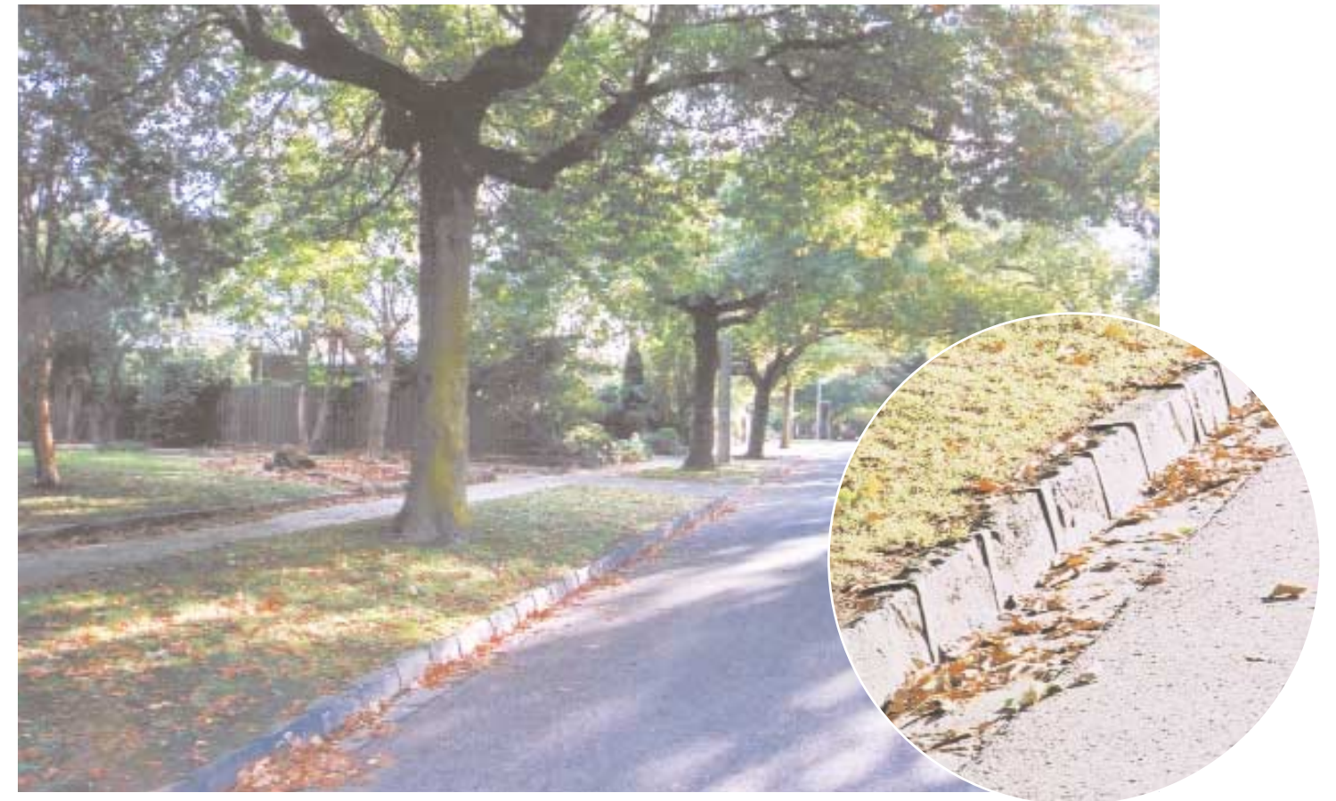
Photo 4. City of Whitehorse, 1 bluestone pitcher channel and kerb, Windsor Crescent, between Elgar Road and Balmoral Crescent, Surrey Hills.
