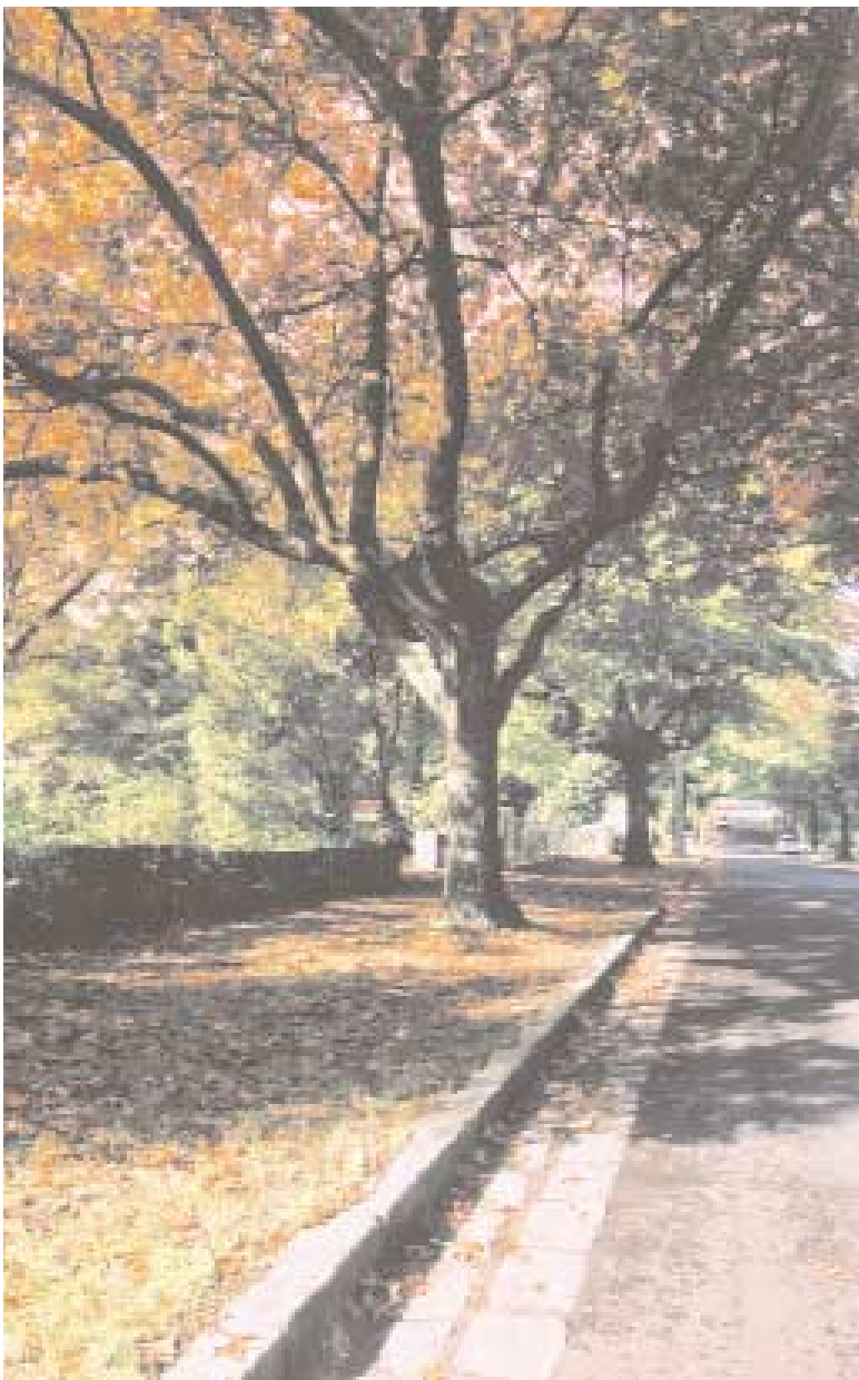
City of Whitehorse, Bluestone Kerb and Channel, Vernal Avenue, between Mitcham Road and Glenburnie Road, Mitcham.
