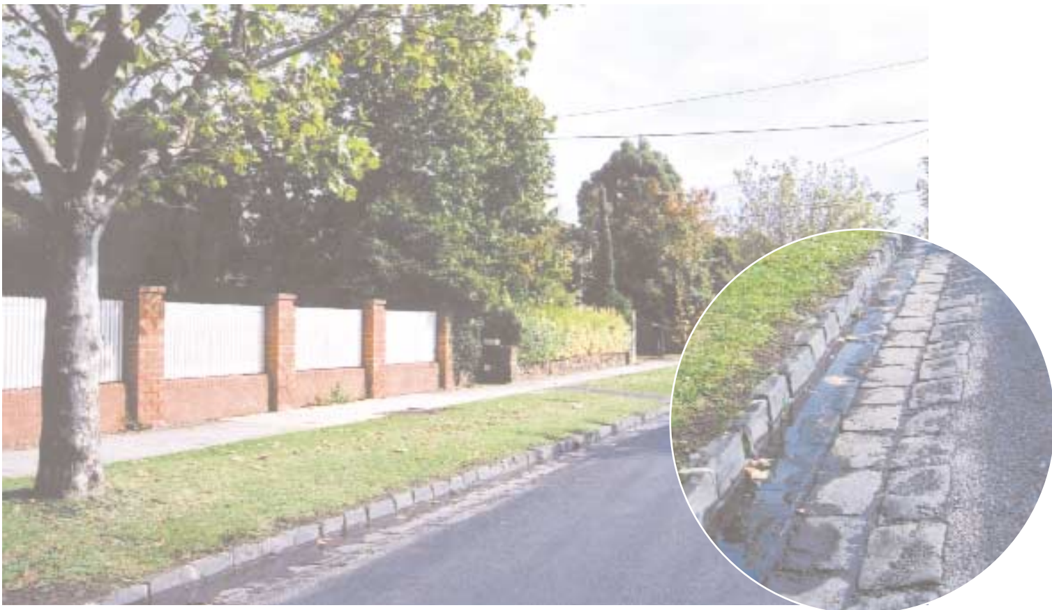
Photo 1. City of Whitehorse, Bluestone Kerb and Channeling, Carrington Road, between Elgar Road and Thurston Street, Box Hill.
