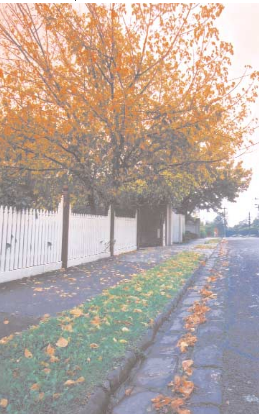
Photo 5. City of Whitehorse, 2 bluestone pitcher channel and kerb, Drewett Street, between Shepherd Street and Erasmus Street, Surrey Hills.
