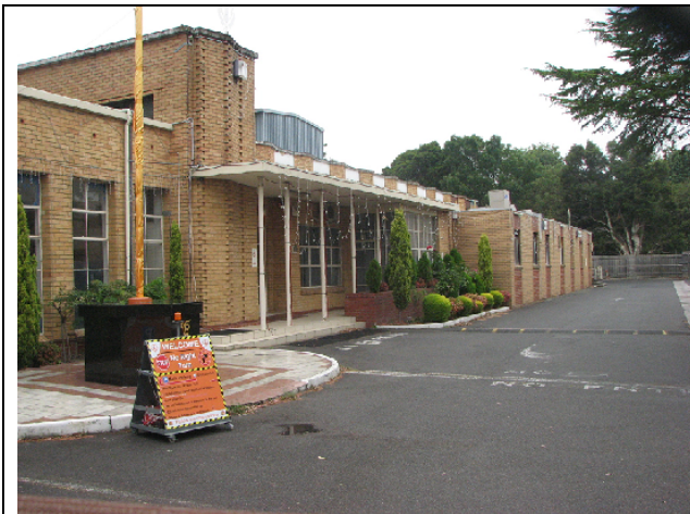
Photograph by Built Heritage, 13 February 2014
