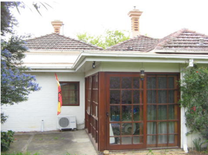
Rear of house Showing full height windows.
