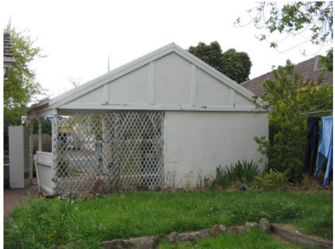
Timber framed garage on south side of house.
