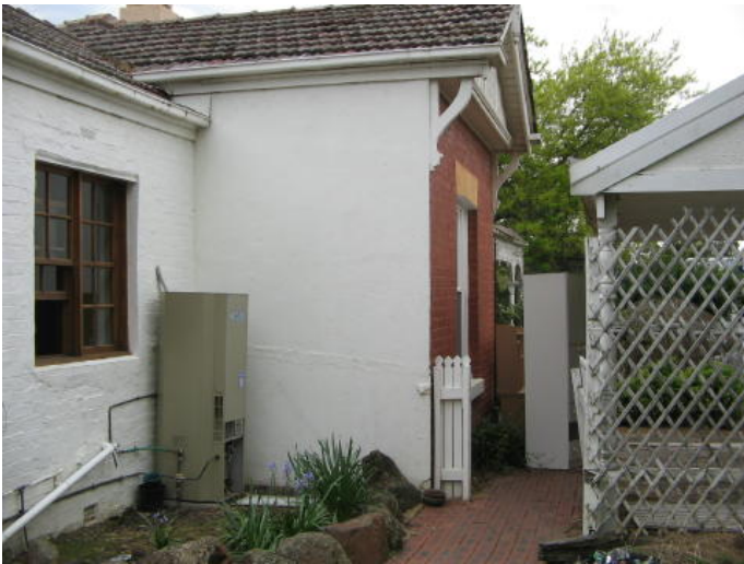
Rear of house and garage
