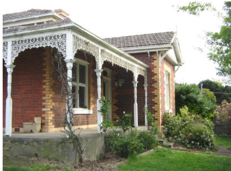
Front of house showing rendered face to verandah & concrete floor. Also showing tiled roof.
