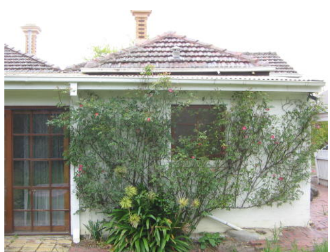
Rear of house showing full height windows.
