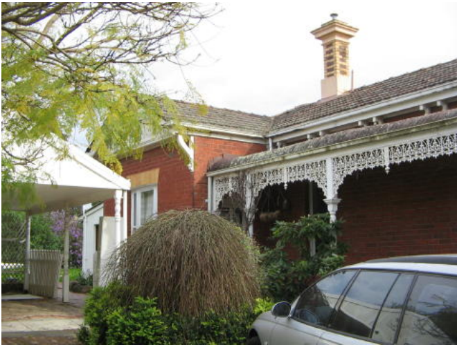
South side of house showing tiled roof.
