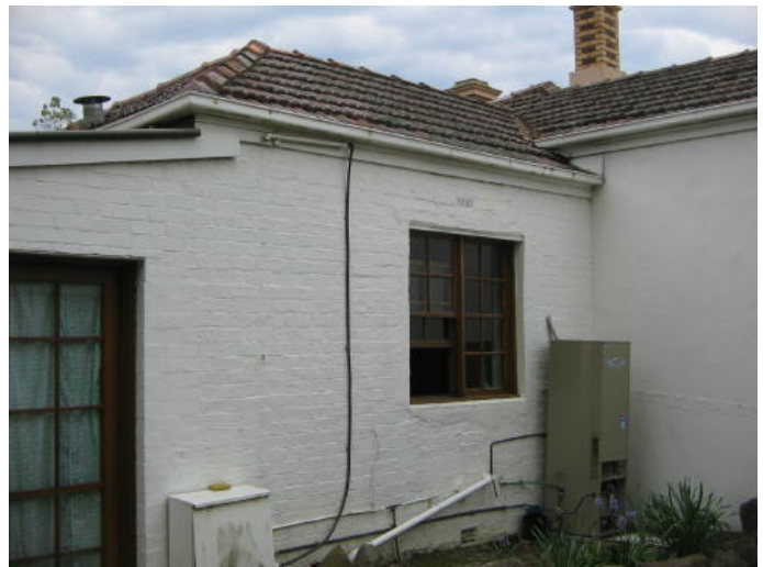
South west corner of house showing gutter heights.
