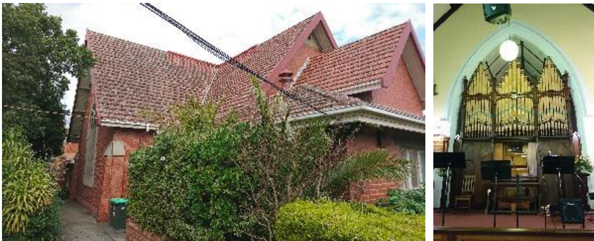
Figure 4: View of the rear (west) of the Main Sanctuary building with the extension housing the Willis Pipe organ to the rhs of the image. Internal image of the Willis Pipe Organ. Source: Trethowan Architecture, 2017.
