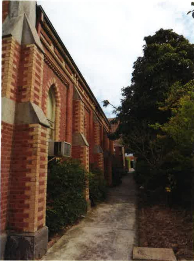
Figure 6. Former Wesleyan Methodist Church – North elevation (part)
