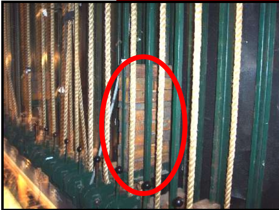
Ropes and counter weights for fly system
