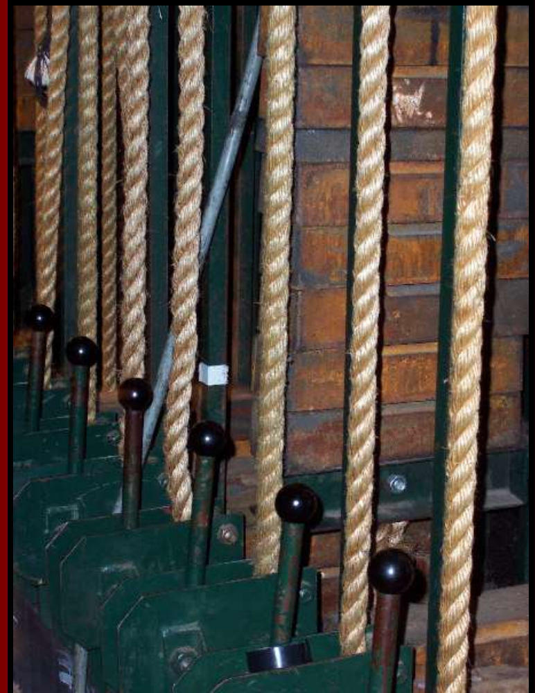
Ropes and counter weights for fly system
