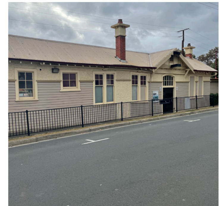
2021 - Mont Albert Station building as it stands today
