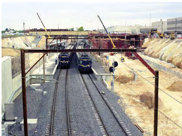
Images: Digging the trench for Box Hill Station (1982)
