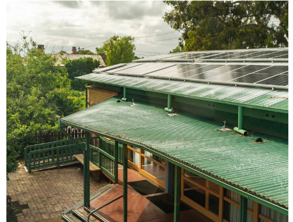
IMAGE: 15KW ROOFTOP SOLAR SYSTEM ON THE BOX HILL COMMUNITY ARTS CENTRE
