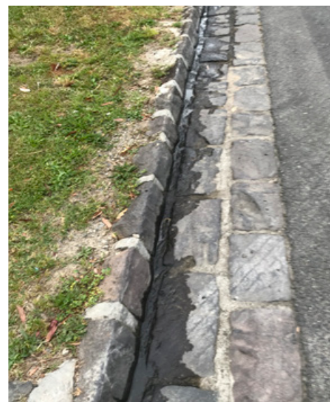
Bluestone Kerb and Channel Existing Railway Road kerb and channel to be retained and reinstated where existing cross-overs are removed
