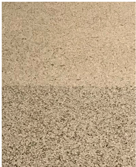
Exposed aggregate insitu concrete paving 2 mixes in alternating bands to match existing Blackburn Station Village improvement works
