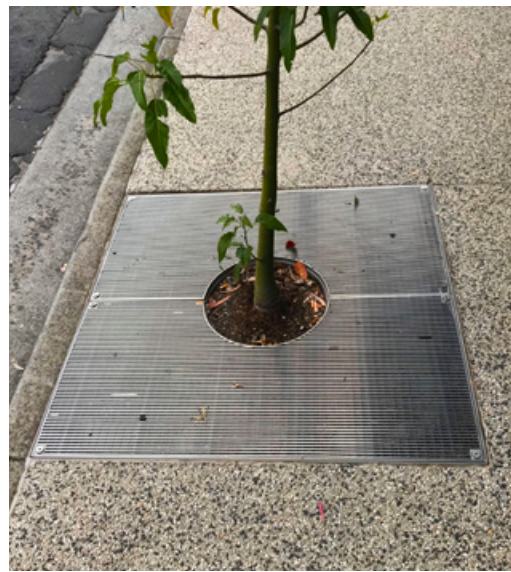
Stainless Steel Tree grate Product and installation detail to match existing Blackburn Station Village improvement works
